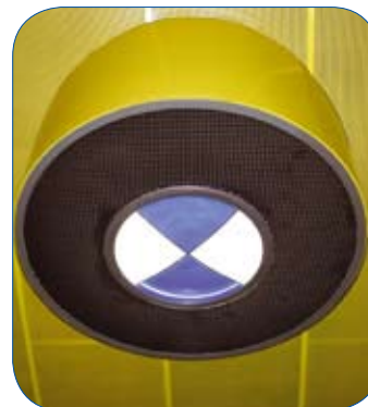
Detail of one of the 1200 Square SunCatcher systems serving the BMW Amenity area
