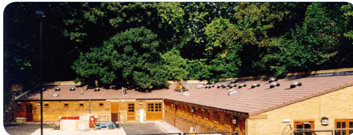
Top: Battersea Park Police Headquarters, where 19 No. 530mm diameter SunPipes were installed to internal cells, corridors and interview rooms.
